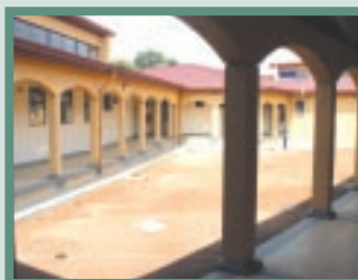
The New Rakai Facility
